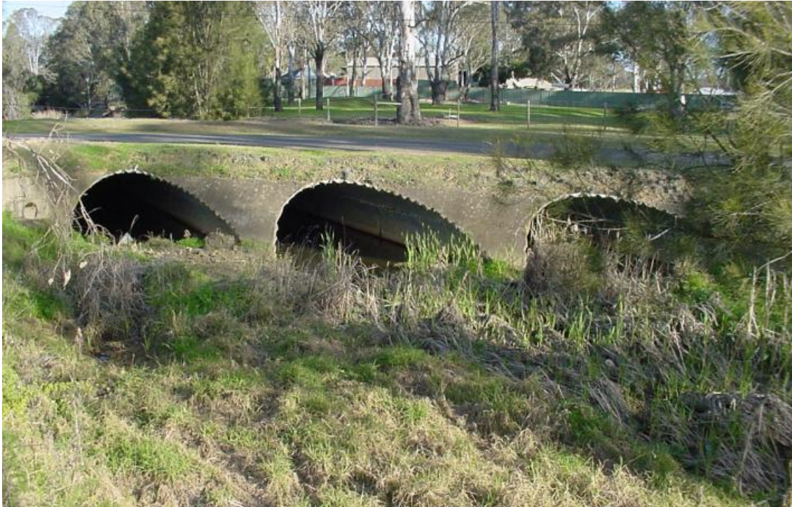
Bonds Creek - looking upstream at 9 th Avenue crossing
